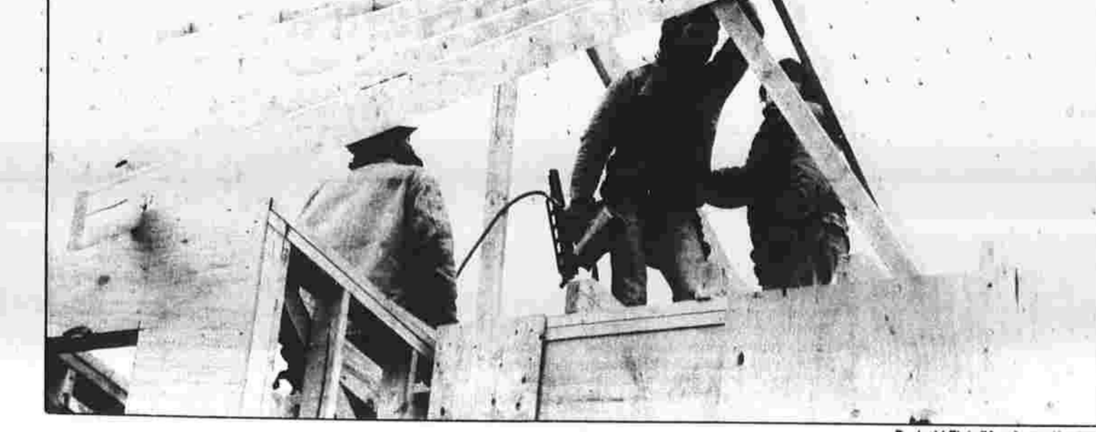
HOUSEWORK — Three construction workers examine their work on one of the new houses under construction Tuesday at Mallard View Homes off Union Street in the North End. From left are Tony Flores, Eric Cox and Joe Crank Jr.
